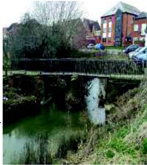
Upstream side showing cutwater on brick pier
