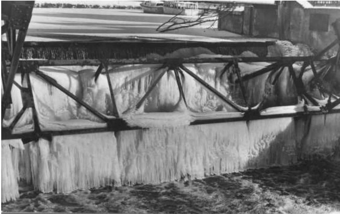
Figure 1 Abbey Mill Sluice Gate 193
