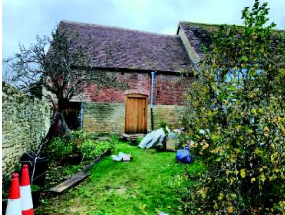
New roof on Barn – 2020
