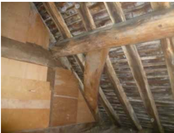
Figure 5: Curved wind braces
