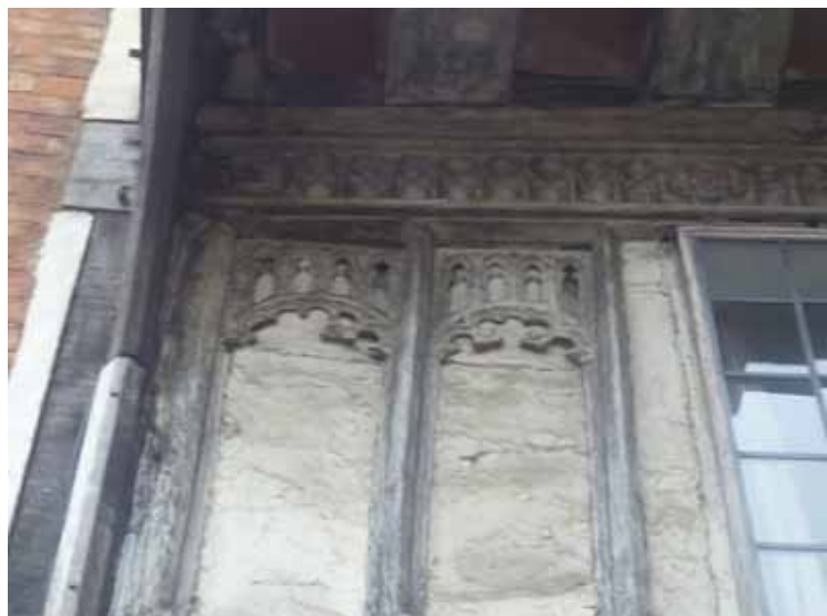
Figure 8: Window tracery with moulded and heavily decorated jetty bressumer above
