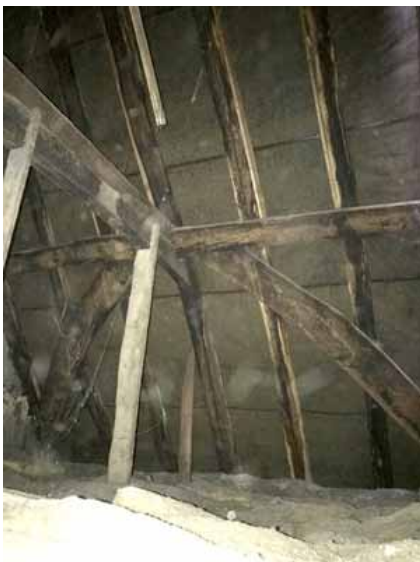
Figure 11: Smoke-blackened roof timbers
