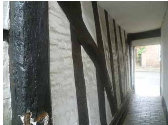
Figure 2: Side passage of 83 Church Street
