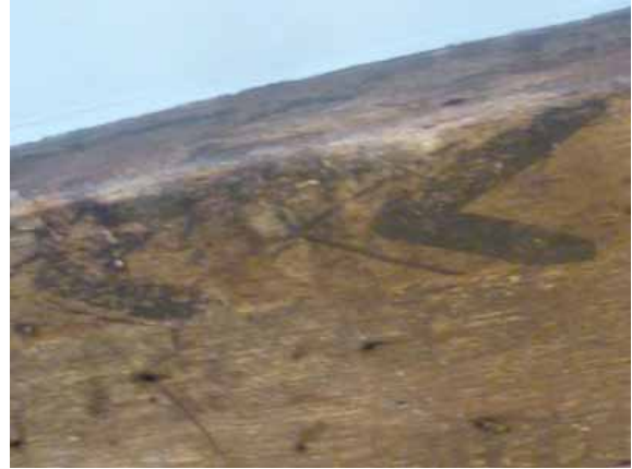
Figure 10: Painted timbers in chevron pattern
