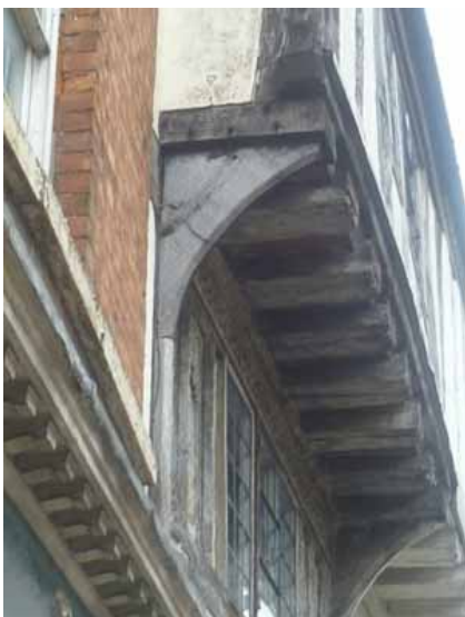
Figure 7: Jetty with simple jetty brackets on buttress shafts
