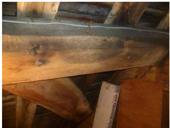
Figure 6: Rafters pegged to purlins
