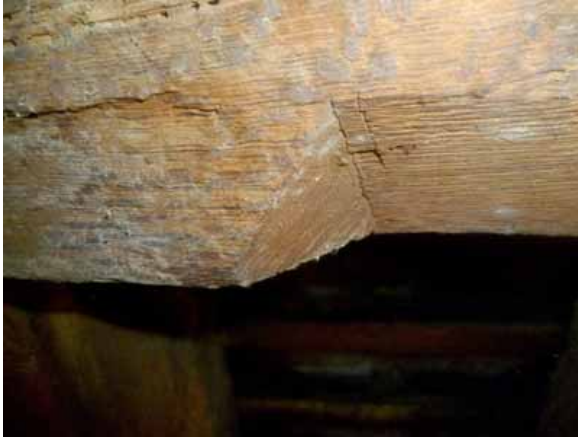
Figure 9: Straight stop
