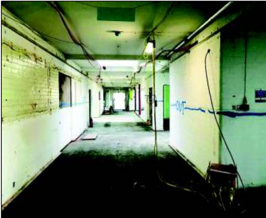
Internal Corridor removed, from Reception.
