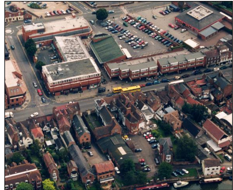
Job Done! A Bird's Eye View of the Shopping Centre In 2003 [TBC]
