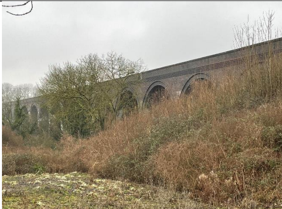
Before climbing to the top of the 50ft/15m high Viaduct
