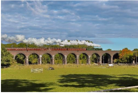
a. GWSR viaduct Appeal
