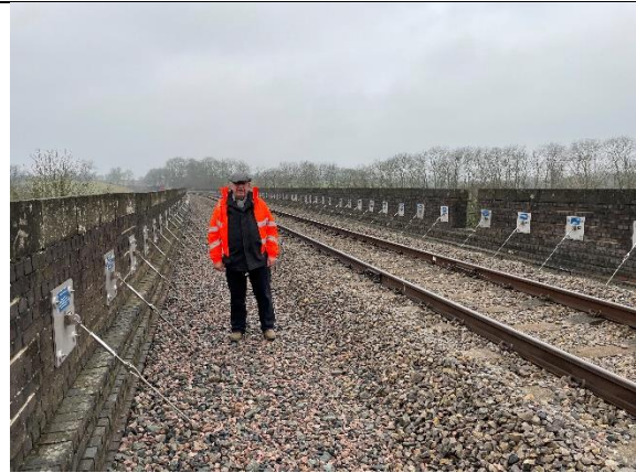
The President flanked by the restraining plates and the plaques along the Viaduct
