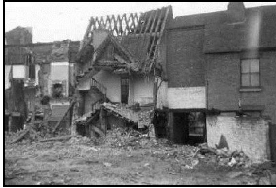
Figure 66: Rear of 84-7 High St., during demolition 1965
