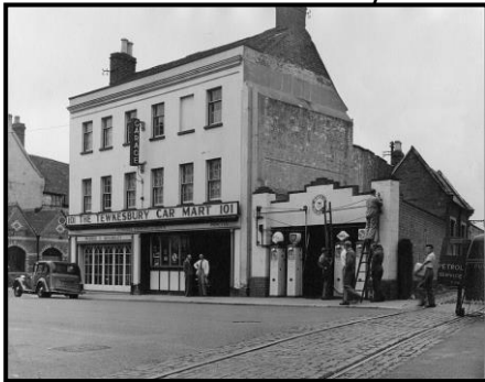
Figure 111: Car Mart and former station in 1951 (MOD)
