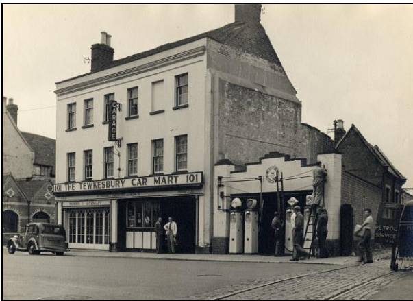
Figure 56: No. 101 High St. The Tewkesbury Car Mart in 1951. This photograph also shows some traces of the 1839 railway station on the gable end of the building including the vertical ashlar strip which used to mirror the one surviving today attached to 103 High St. The gabled platform shelter is also seen as are the railway lines, set in cobbles, crossing the High St. towards Healings Mill . (TBC)
