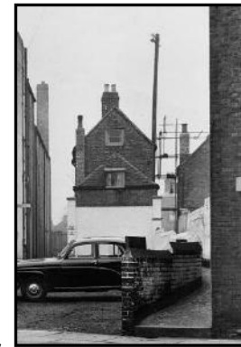
Figure 44: close up of Bishops Alley before demolition. (TBC)
