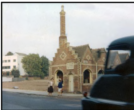
Figure 91: 1-2 Market Shops with outsize chimney (P. Preston)
