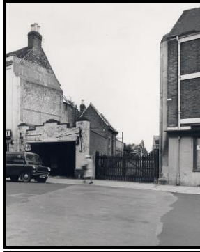
Figure 109: Station remains in c 1960 with platform occupied with Car Mart petrol pump. (MOD)
