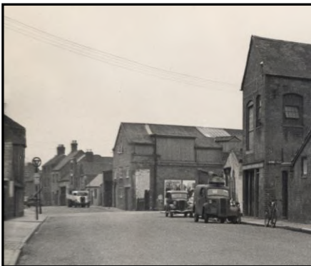
Figure 100: looking south in 1949 (TBC)
