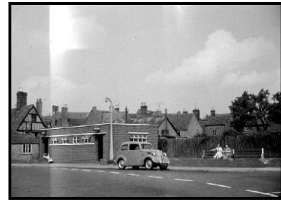
Figure 101: Sun St. public toilets in c1960 (Butwell)
