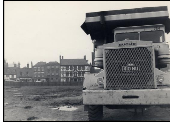
Figure 16: Demolition contractor's earth mover at Bishops Walk c 1965. (TBC)
