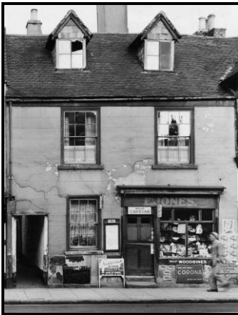
Figure 76: 89 High Street showing also Glovers Alley (MOD)
