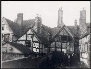
Figure 98: Rear of Mayalls Court & Glovers Alley (TBC)
