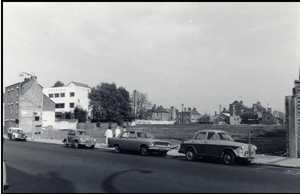
Figure 15: Bishops Walk site c.1965, only the Sabrina and numbers 83 and 84 High St survive. (TBC)
