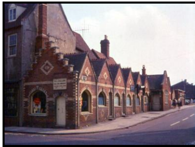
Figure 89: Market Shops before Demolition. (Butwell)
