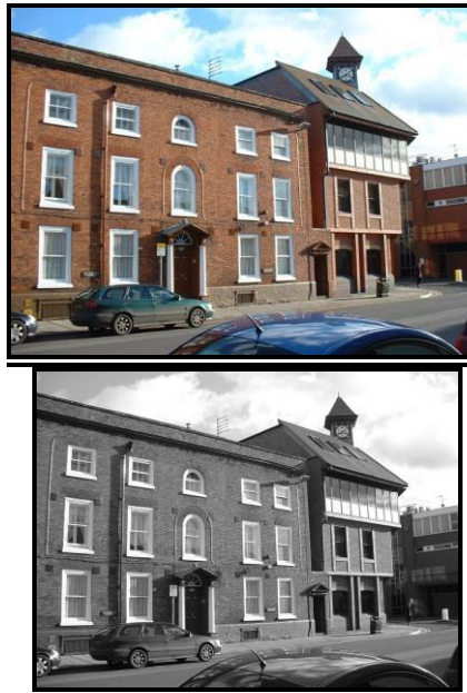
Figure 36: The site today - The Library and the Modern Sun Street (Dixon)
