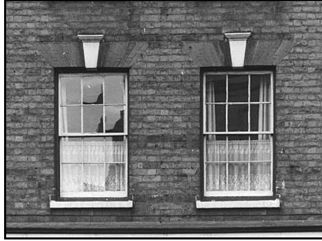
Figure 10: Surviving Georgian glazing bars. (MOD)
