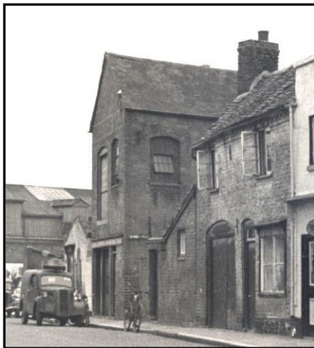
Figure 13: Tewkesbury Engineering Company, Oldbury Rd., 1949 (TBC)
