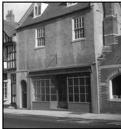
Figure 14: the shop front installed in 91 High St. c.1952 (TBC)
