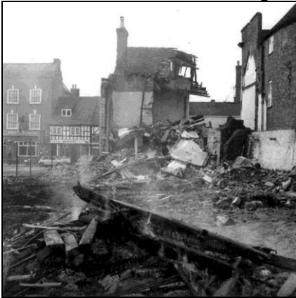
Figure 18: Demolition of 80 High St. (Tewkesbury Library).
