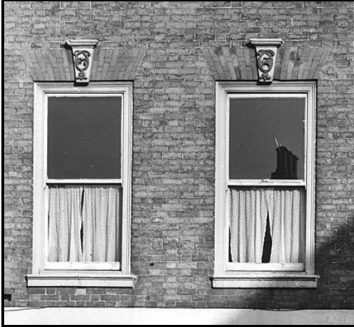
Figure 9: Lost Georgian glazing bars. (MOD)
